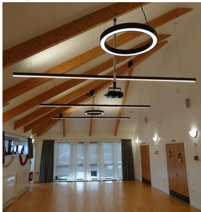
The new energy efficient LED lighting scheme
